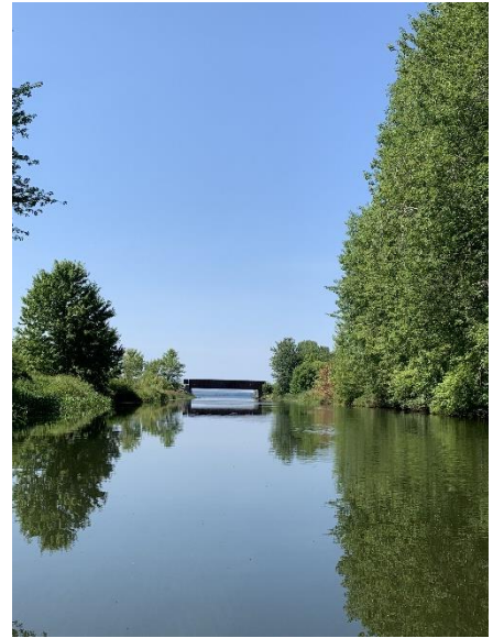
Sandy Stream & Train Trestle (Photo Credit: Alan Burton)
